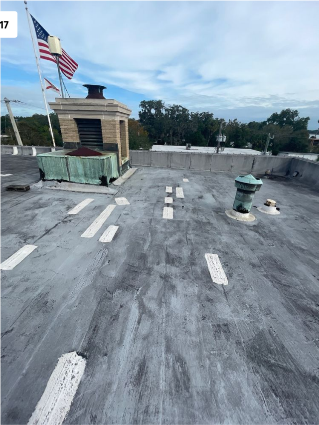
Previous silicone repairs
