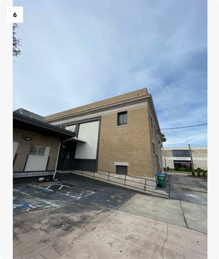
A/C side and back parking lot side
