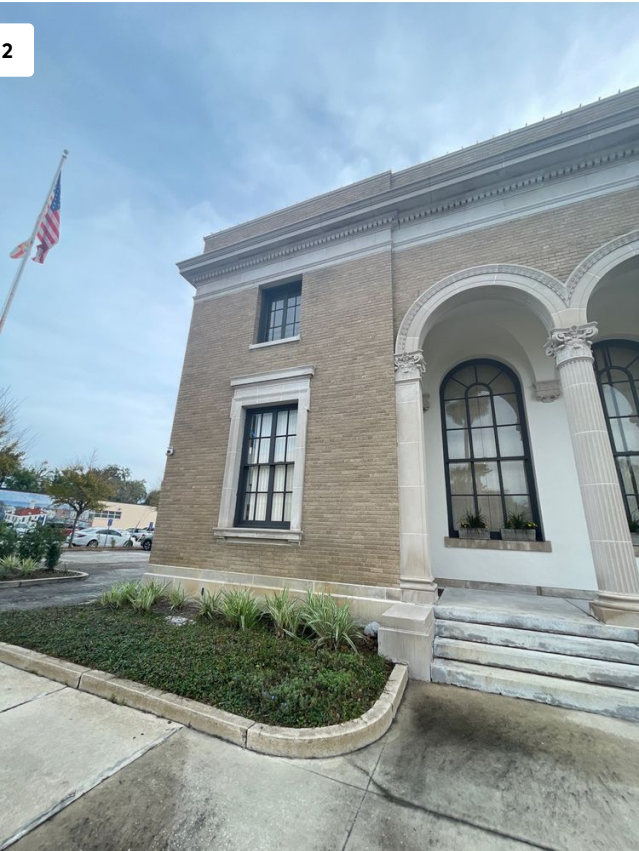
Main Entrance and Back Parking Lot
