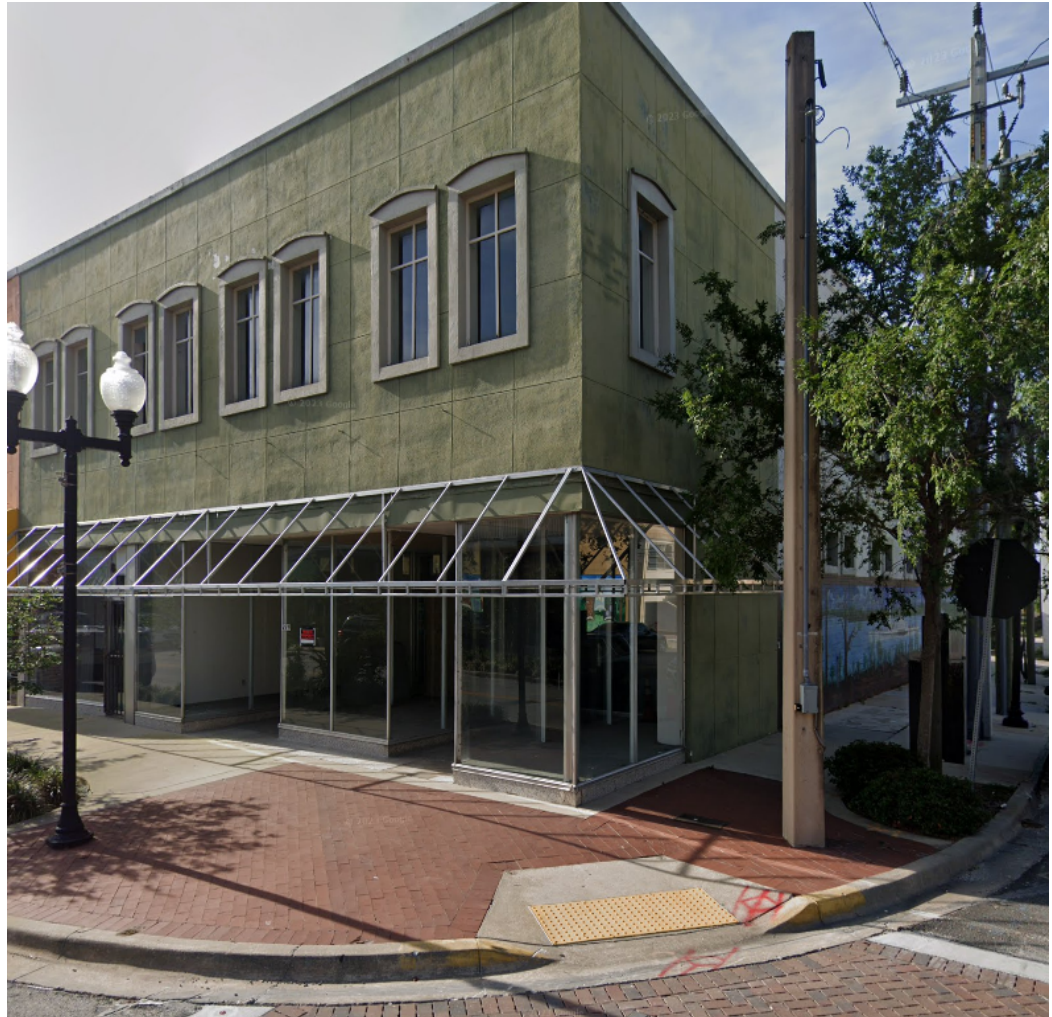
Figure 3: View of 229 St. Johns Ave from street; photo by Google, Apr. 2023.
