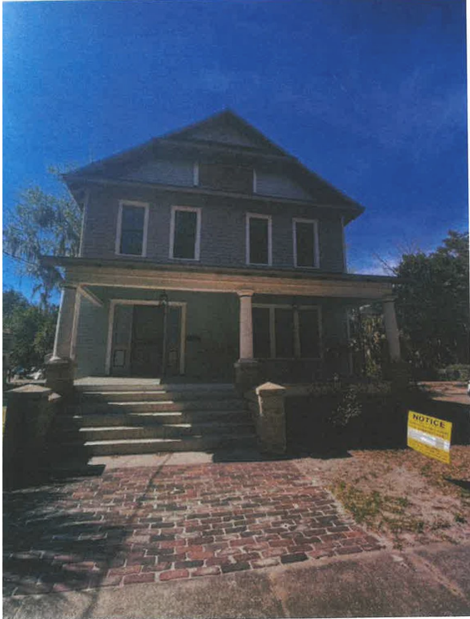
Figure 2: Current picture of structure.
