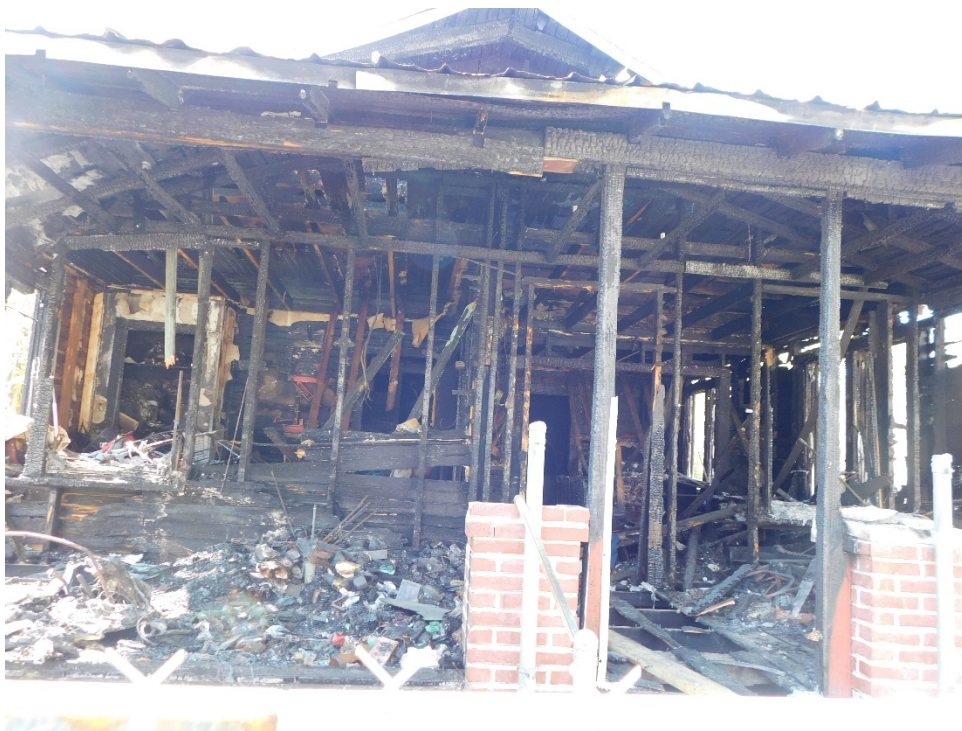
Pre-demolition (D. Green)
