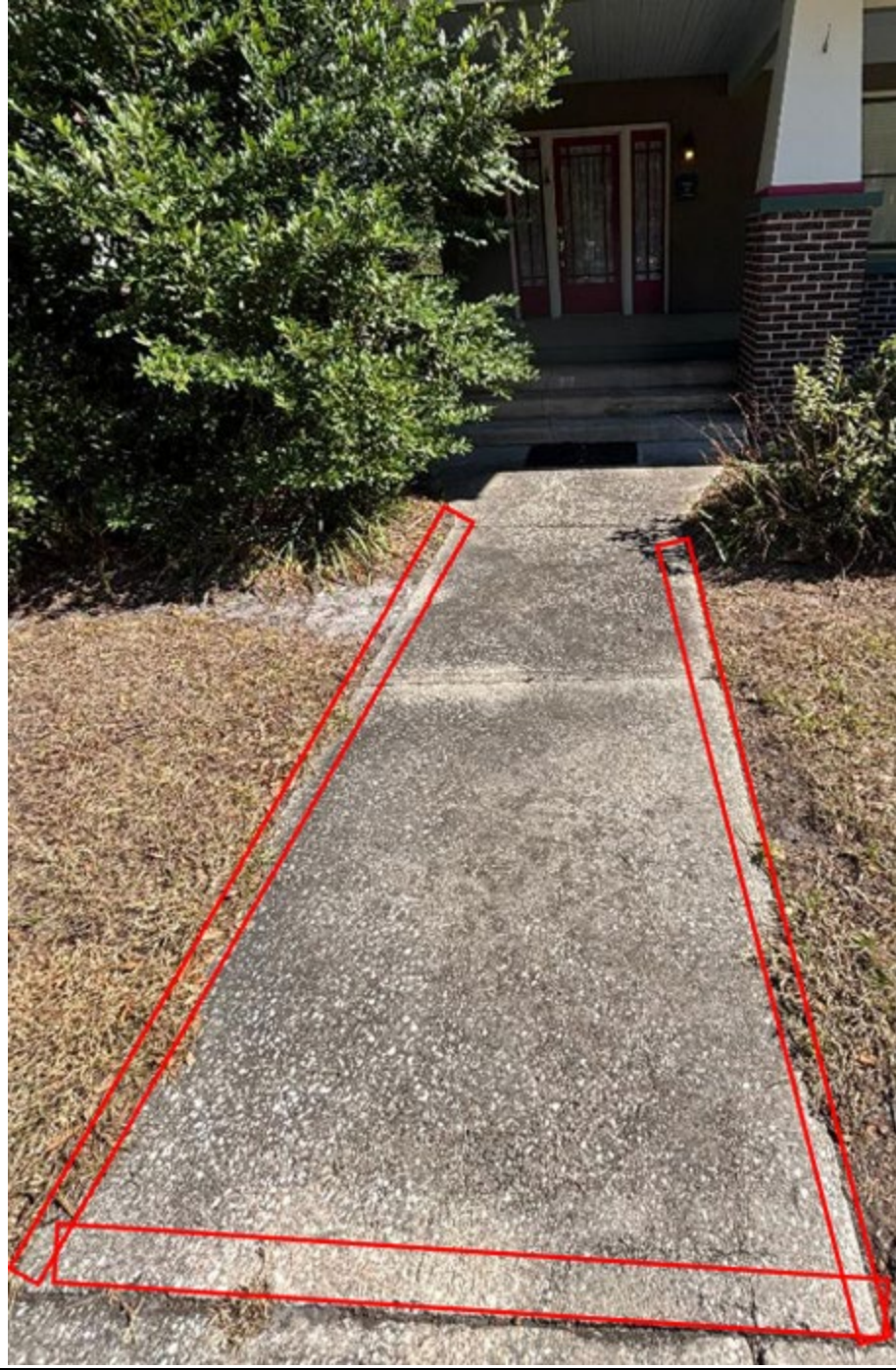
Figure 10: Resurface front walkway.
