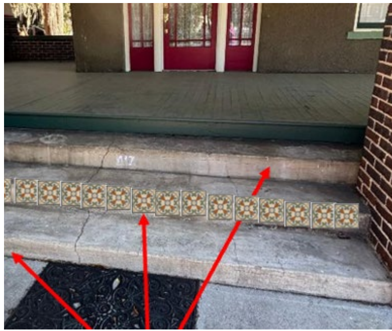
Figure 11: AI image of tile on front step risers.
