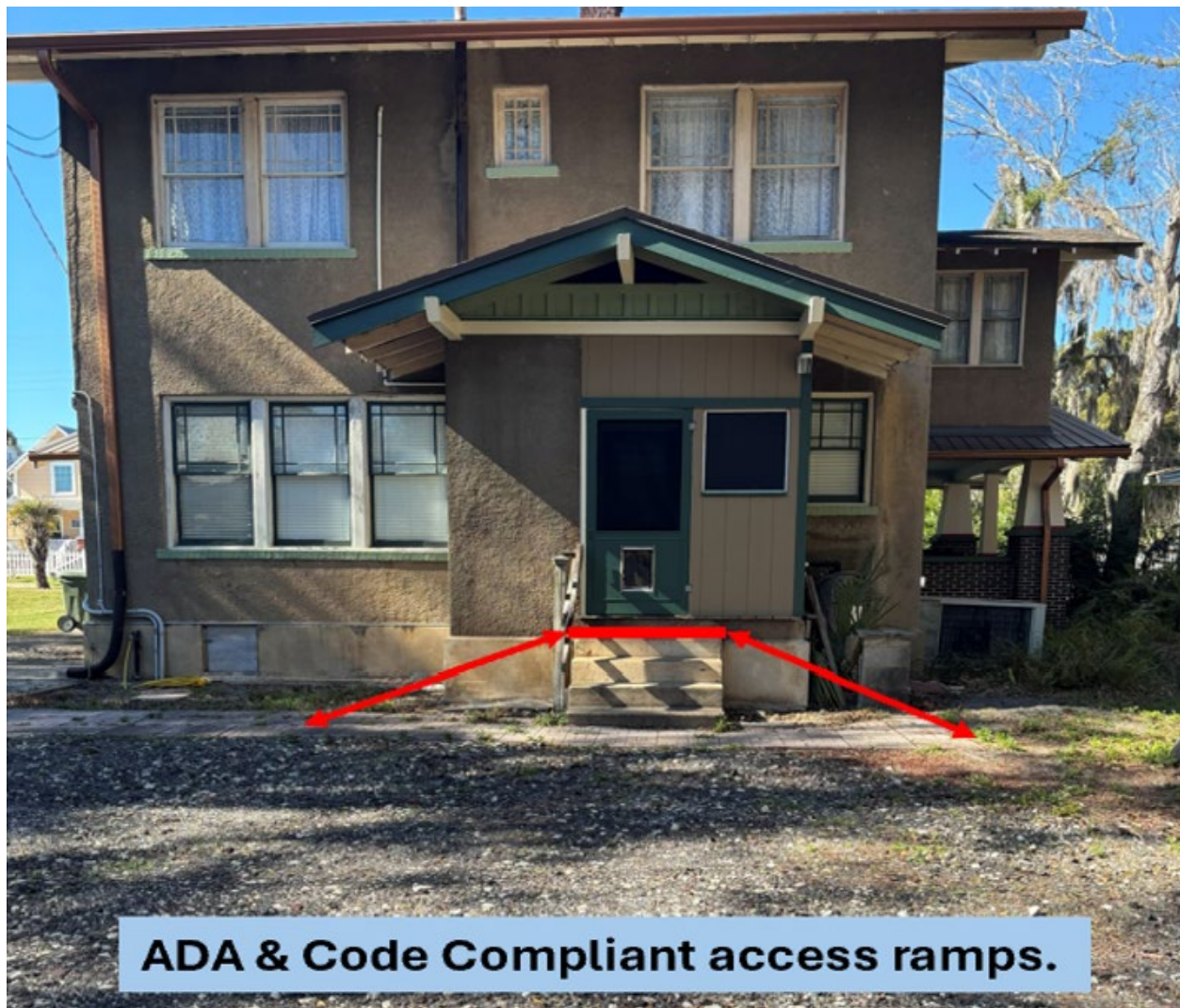
Figure 8: Ramp over back stairs.
