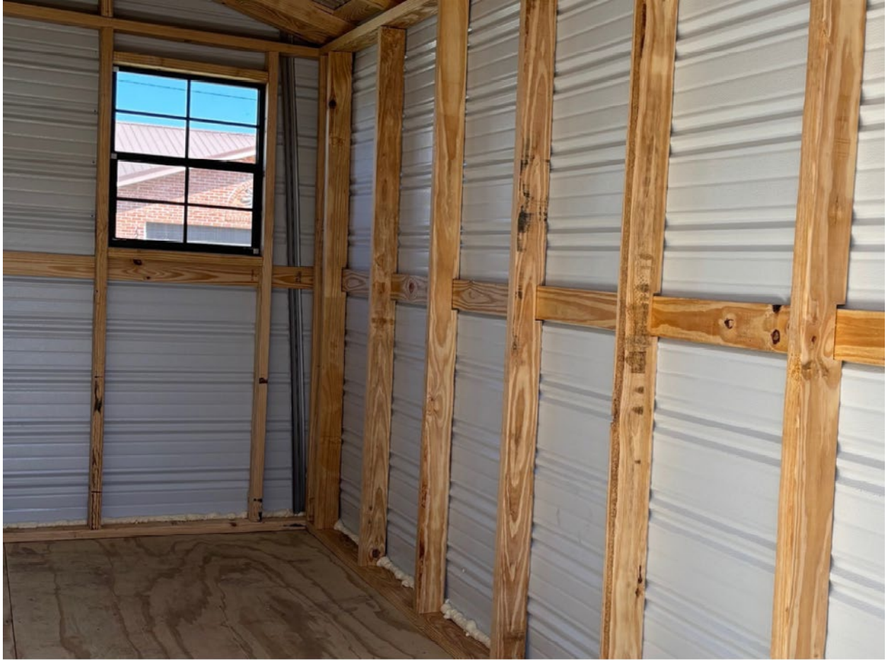
Figure 5: Interior of shed.
