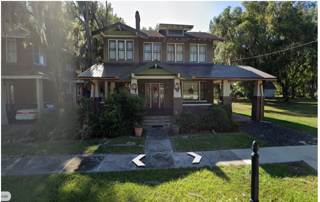
Figure 2: Current picture of structure.
