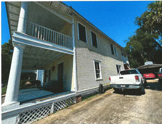
Figure 2: Current photos of house railings, stairs, and porches.
