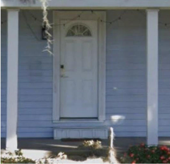
Figure 3 Photograph of the existing front door.
