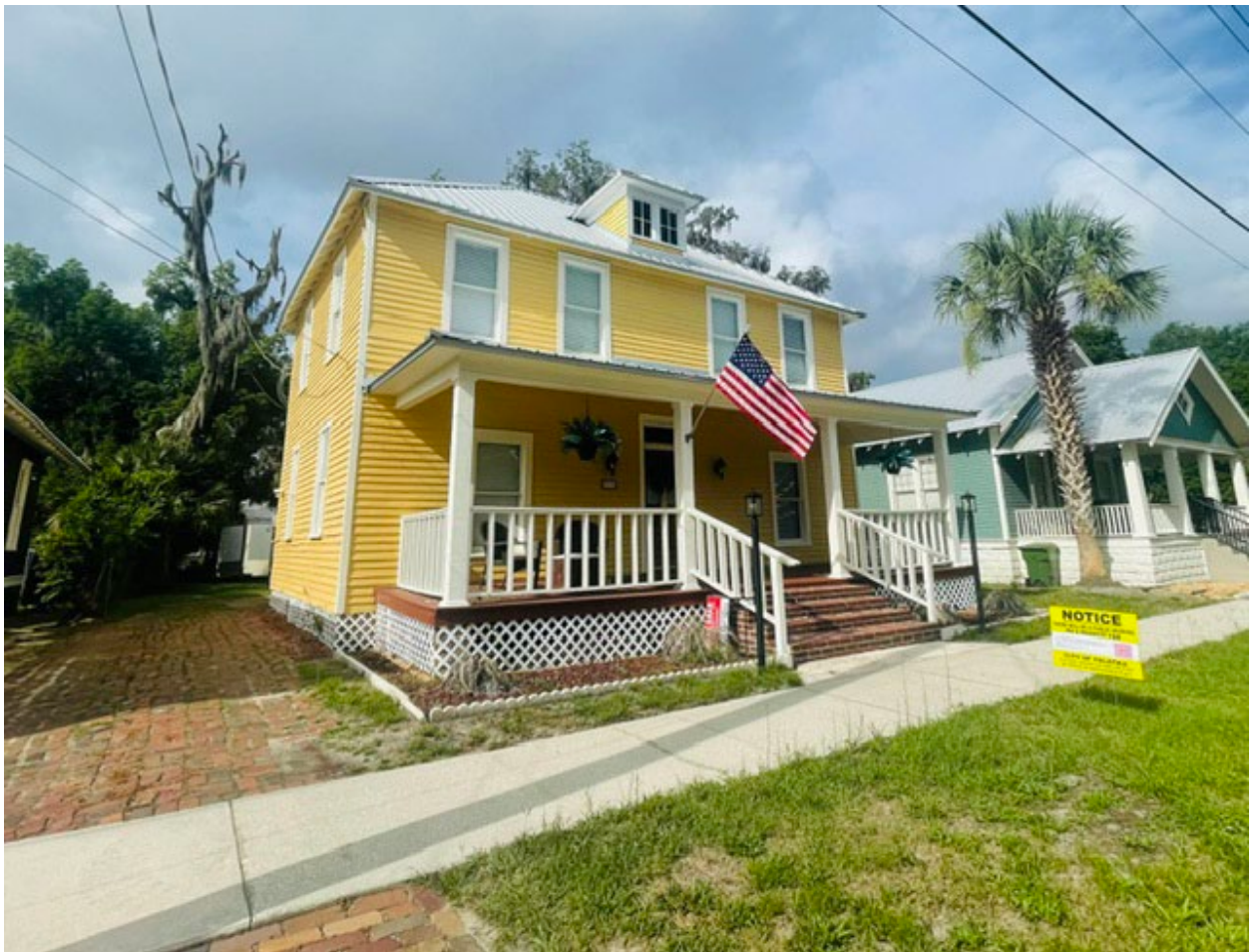
Figure 2: East side of structure.
