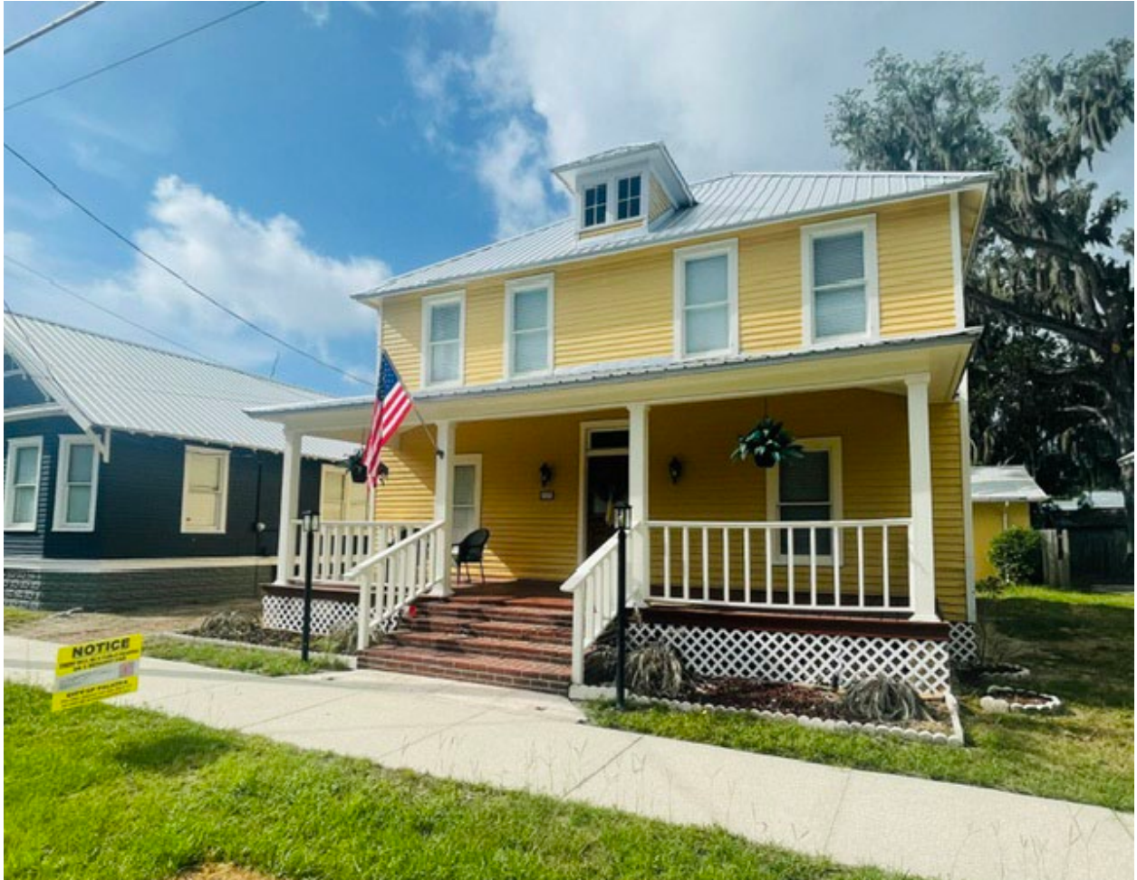
Figure 3: West side of structure.
