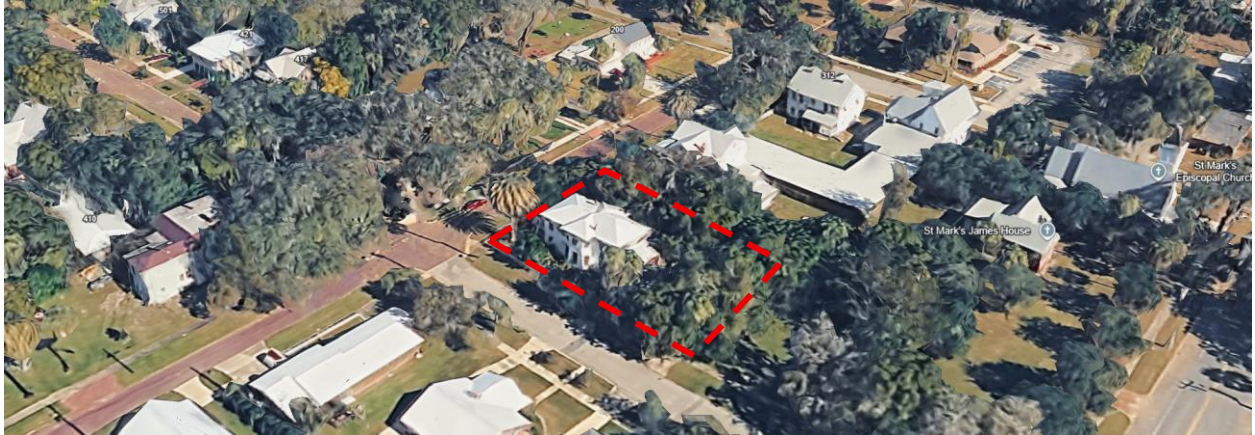
Figure 1 Aerial view of the North Third and Madison Street area (source: Google Earth)
