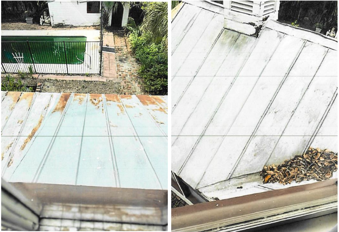
Figure 3 Above: photographs of the metal roof that will be replaced over the porch. Below: Image of the metal roof that is in good condition on the house.
