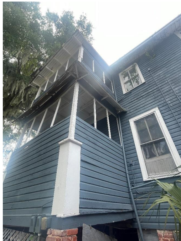
Figure 10 & 11: Rear balconies with \frac{3}{4} wall to be replaced with railings.
