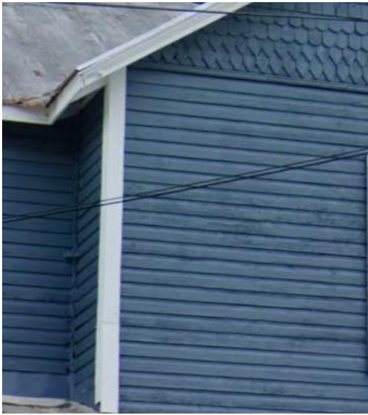
Figures 6 & 7: Existing clapboard and the pine replacement boards.
