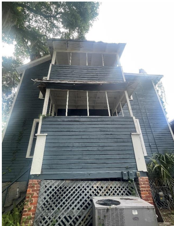
Figure 10 & 11: Rear balconies with \frac{3}{4} wall to be replaced with railings.
