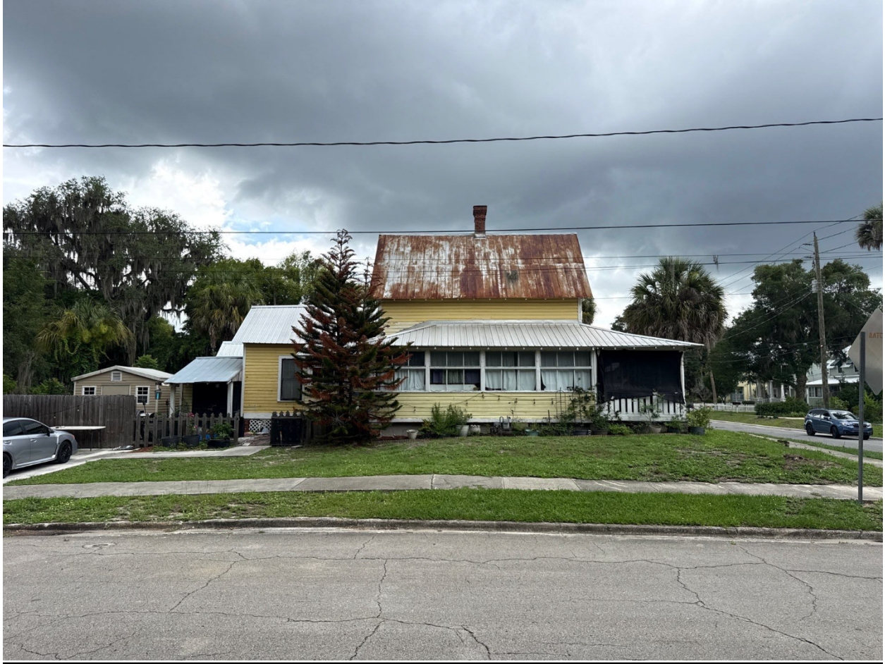
Figure 4: View from Morris St.
