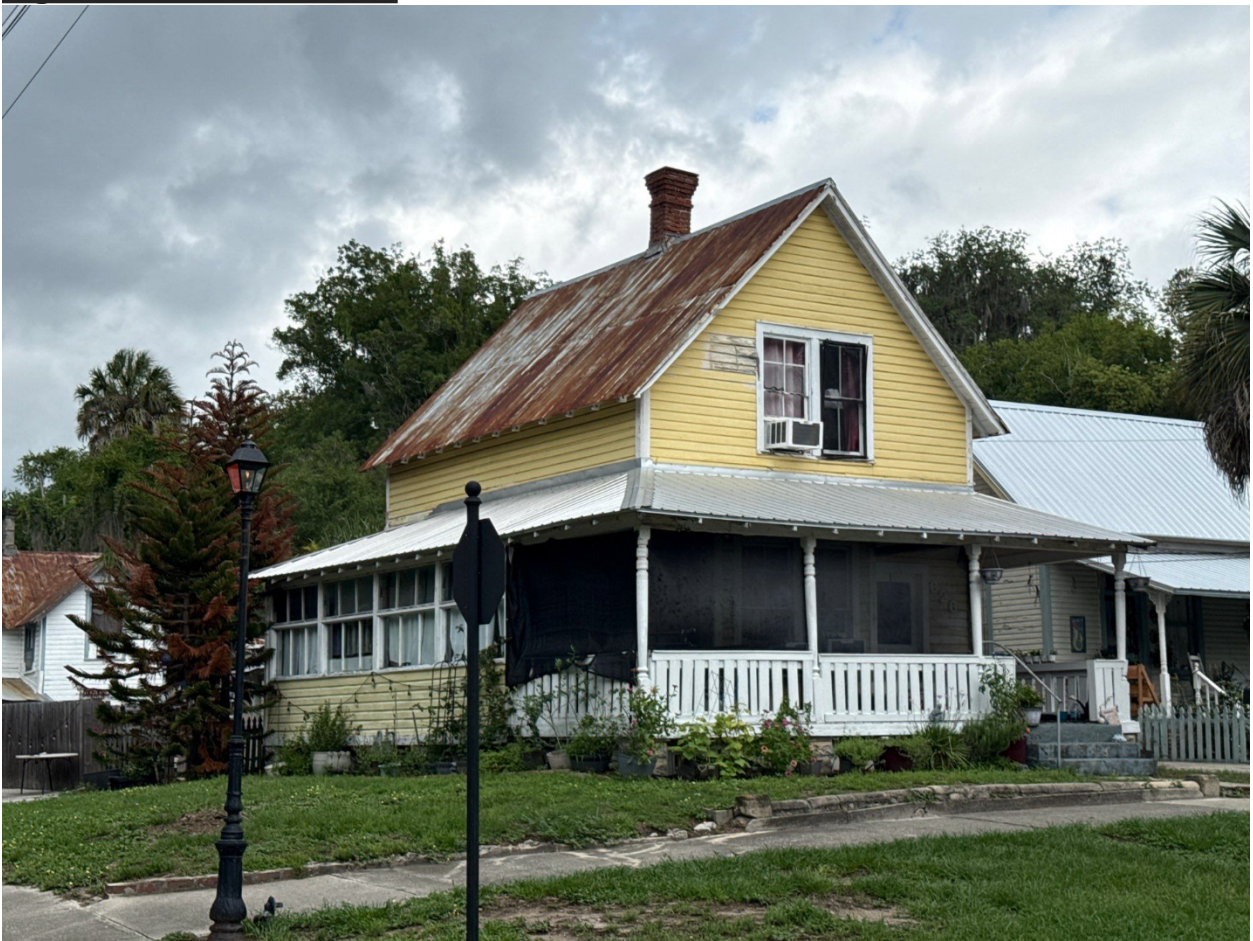
Figure 3: View from the corner.
