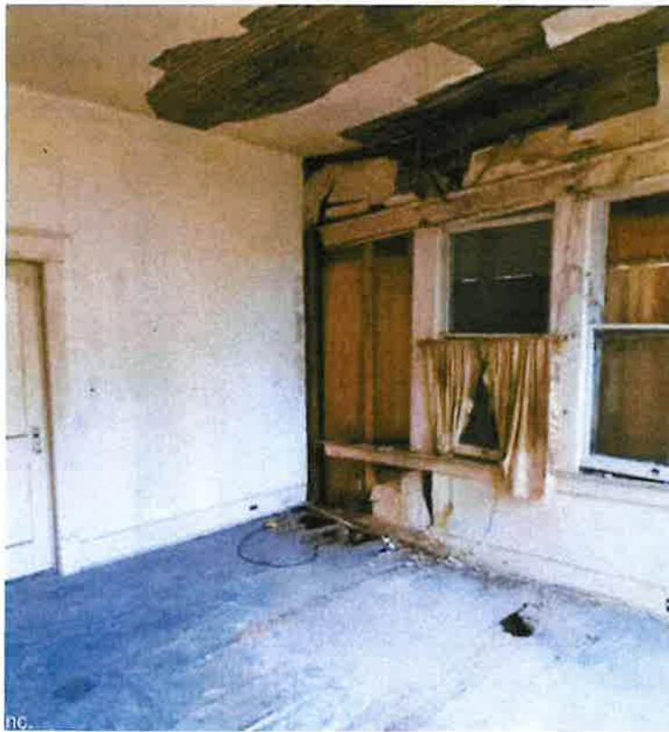
The "bad" section 2. floor
