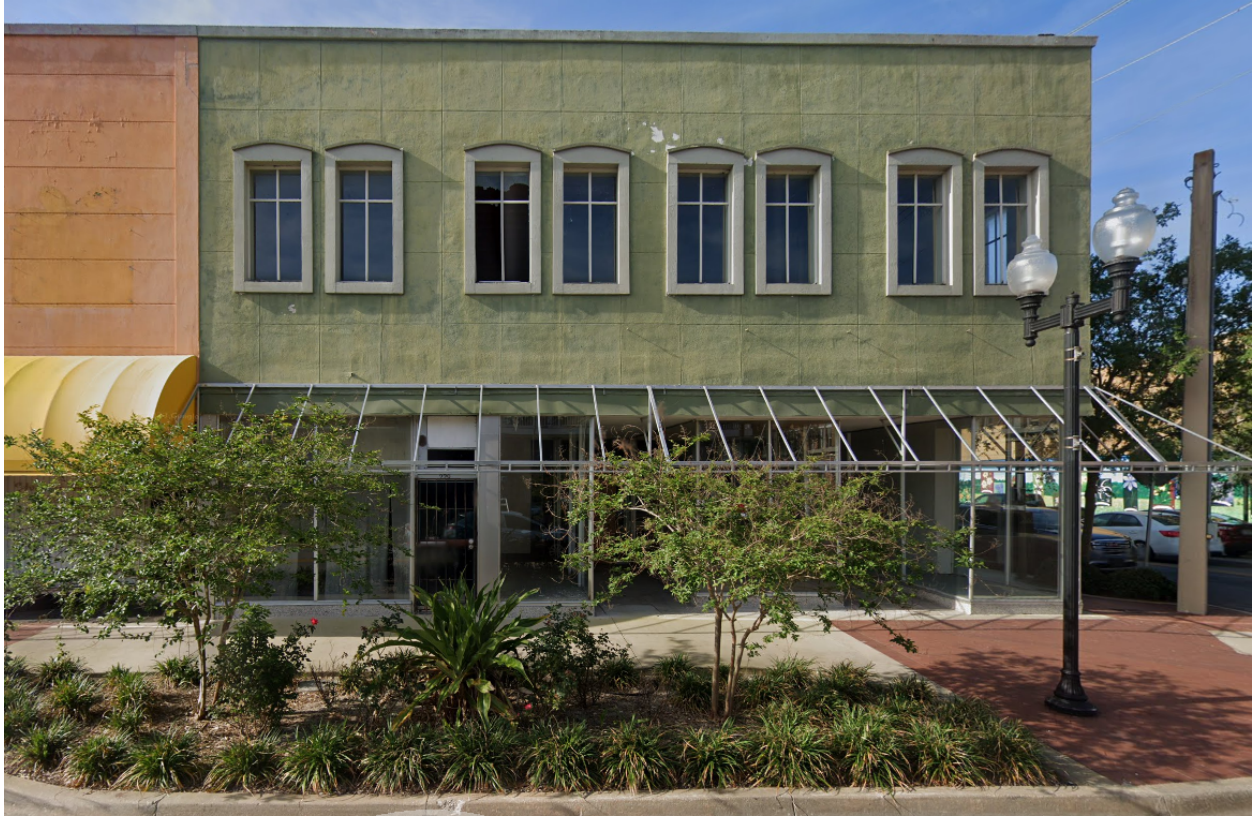
Figure 3: View of 229 St. Johns Ave from street; photo by Google, Apr. 2023.
