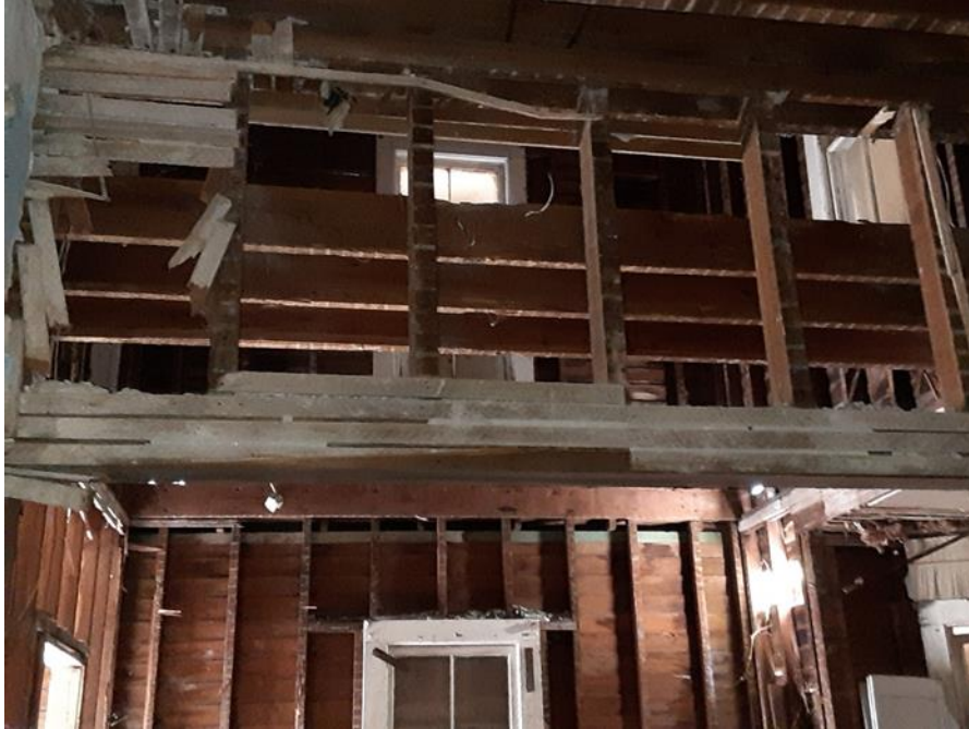
First and Second Floor Wood Framing: The exposed members appear to be in good condition.
