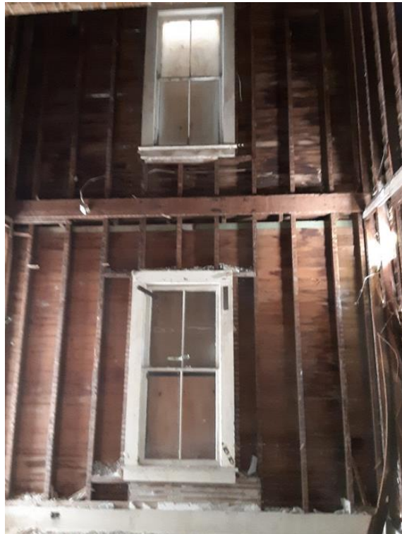
Exterior Wall Framing: Balloon Framing; Structural Members in good condition; some darkened/stained siding.
