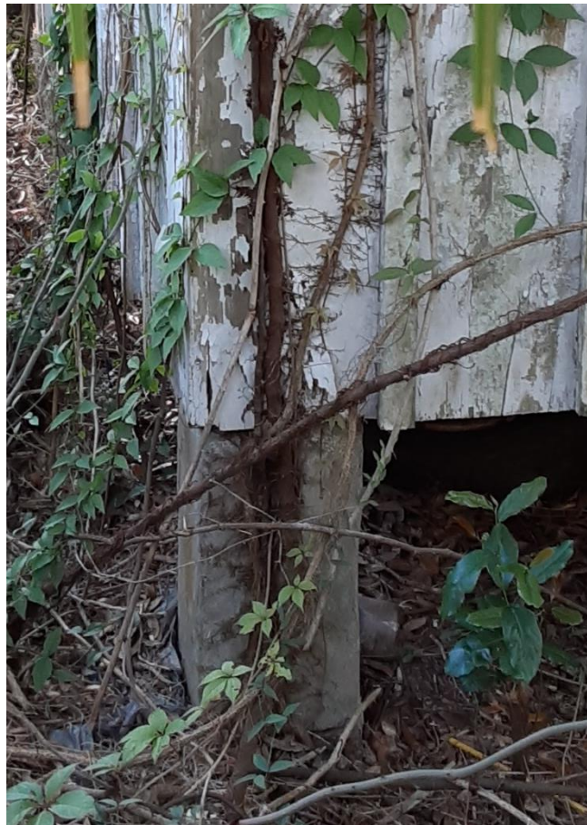
Pier: Rear Left (North West) Corner
