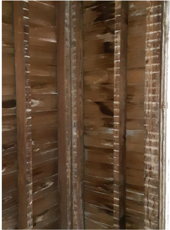
Corner Framing: Studs in good condition; 2x4 actual size studs.
