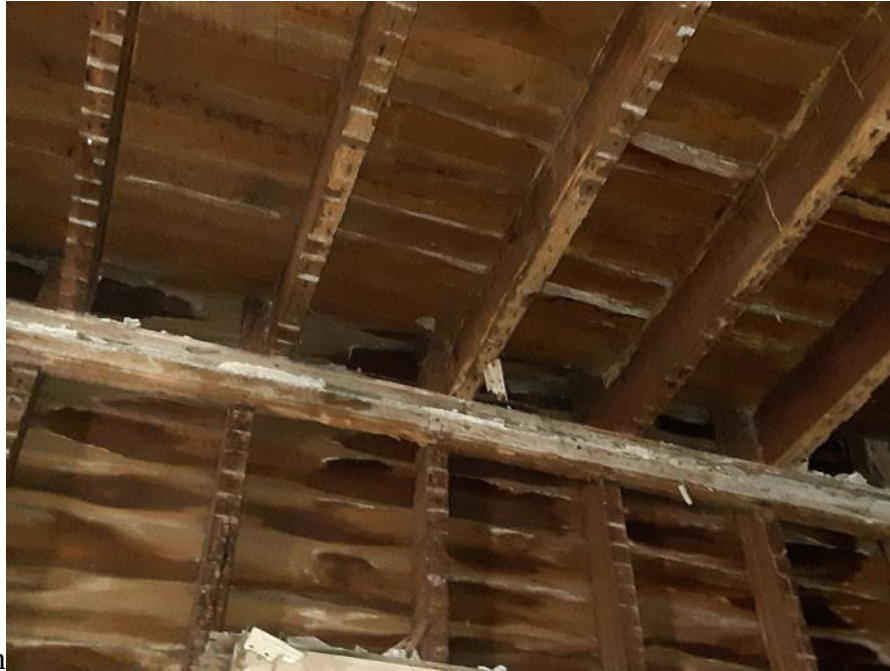
Balloon wall studs and second story floor joists
