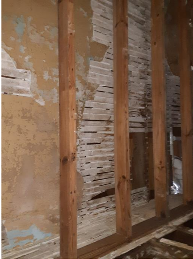
Interior Wall: Studs in very good condition.
