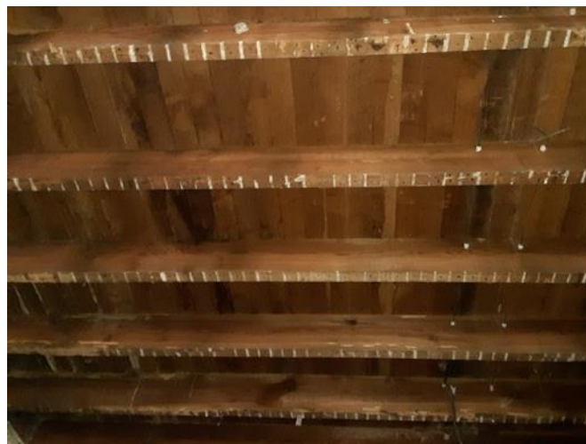
Ceiling/Floor Joist and Subfloor for Second Floor: Structural Members in Very good Condition.
