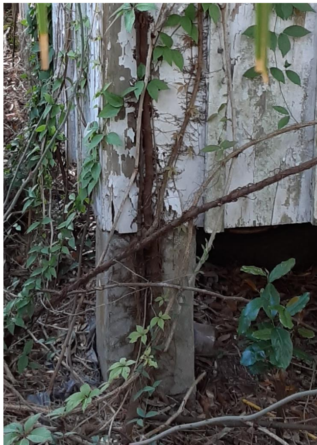
Pier: Rear Left (North West) Corner
