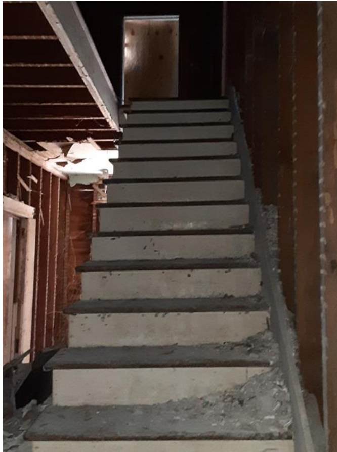
Staircase: Structural sound and fully Intact
