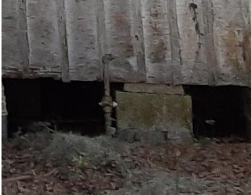
Pier: Left Rear (West-North) room along back wall.
