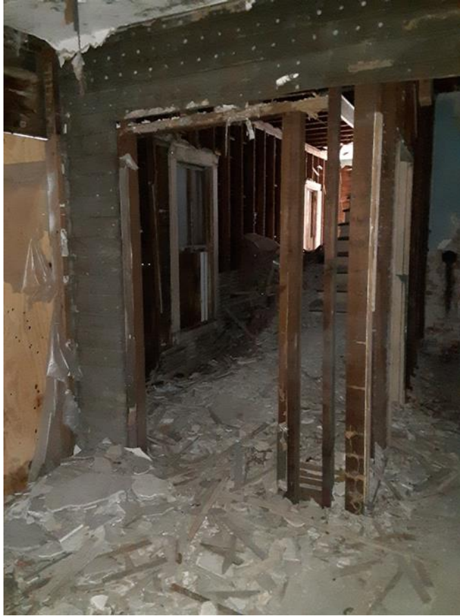
Interior Wall and Door Framing:
