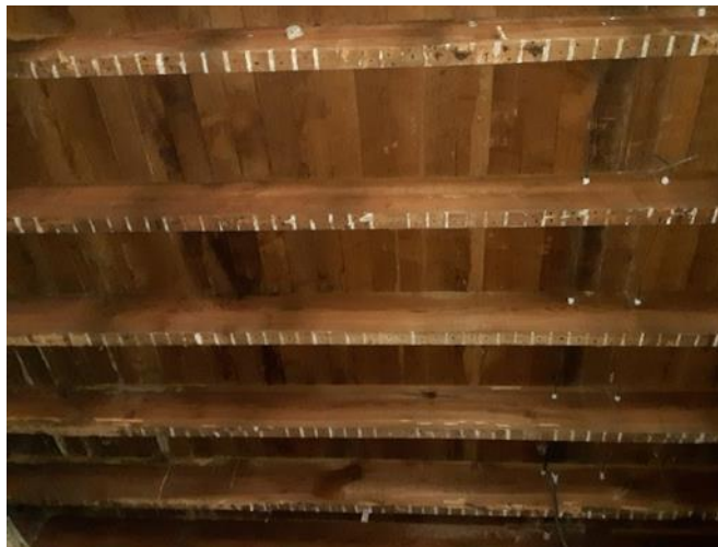
Ceiling/Floor Joist and Subfloor for Second Floor: Structural Members in Very good Condition.
