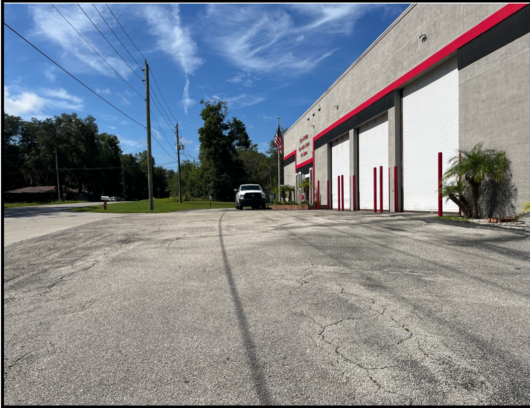
Southerly view of proposed permanent easement area. (Photo #1)
