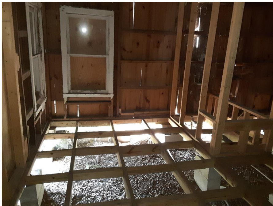
Left Rear (West-North) Room: Wall and Floor Repair
