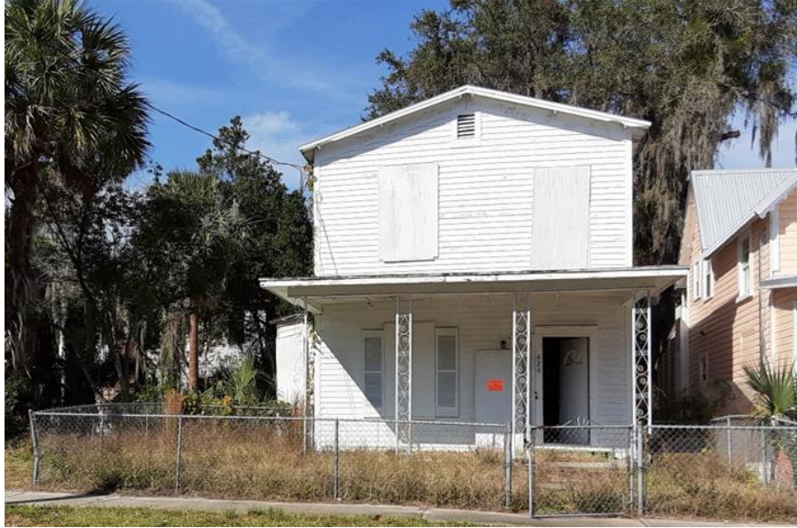
Front (South) View: Overgrown vegetation and relatively flat lot.
