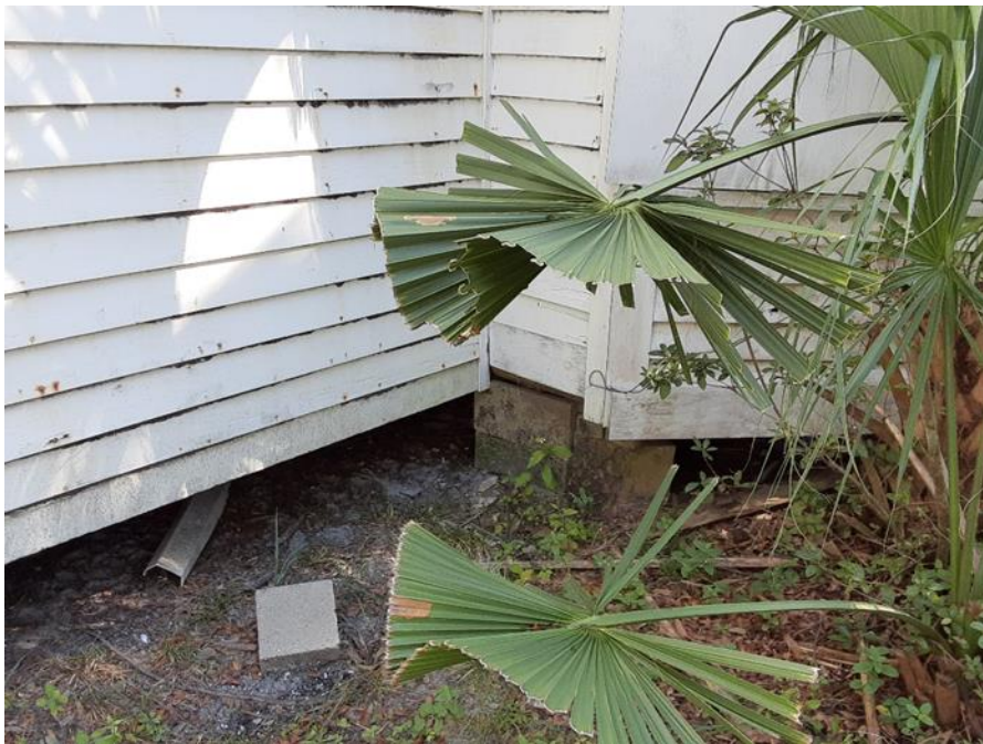
Pier Concrete block
