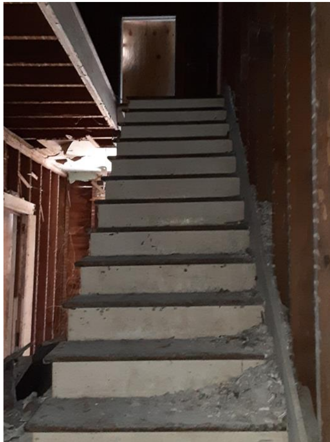
Staircase: Structural sound and fully Intact
