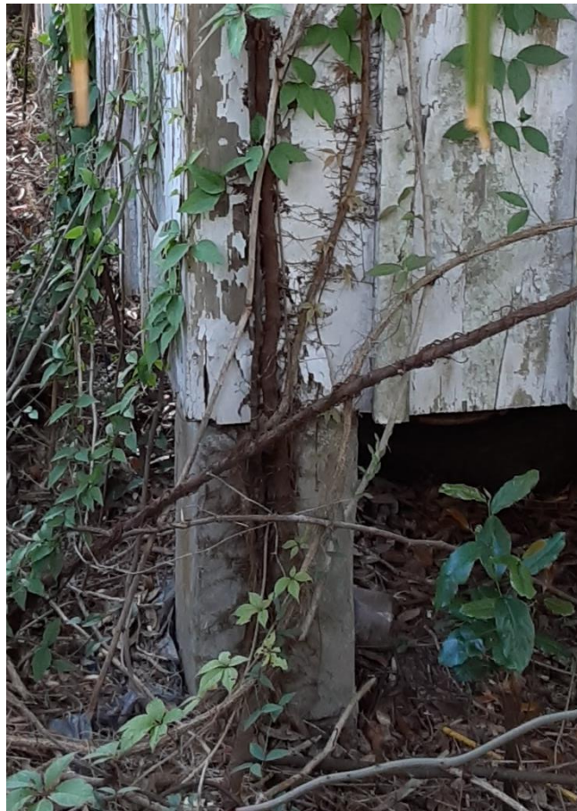
Pier: Rear Left (North West) Corner
