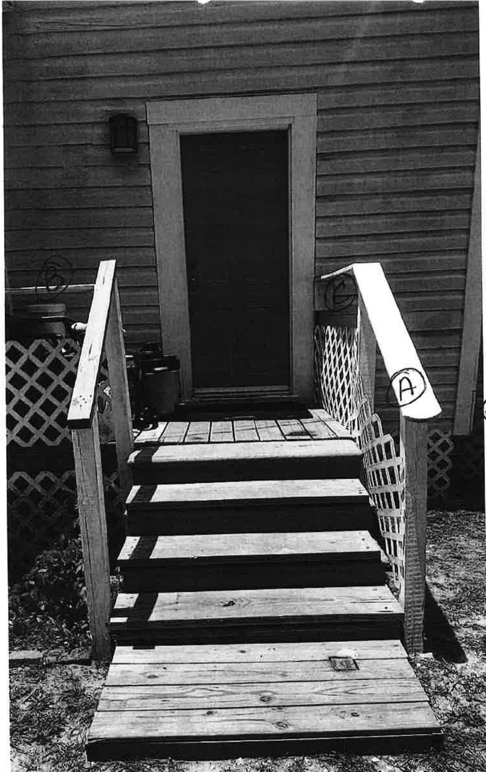
Figure 4: Existing Side Porch 420 Kirby St
