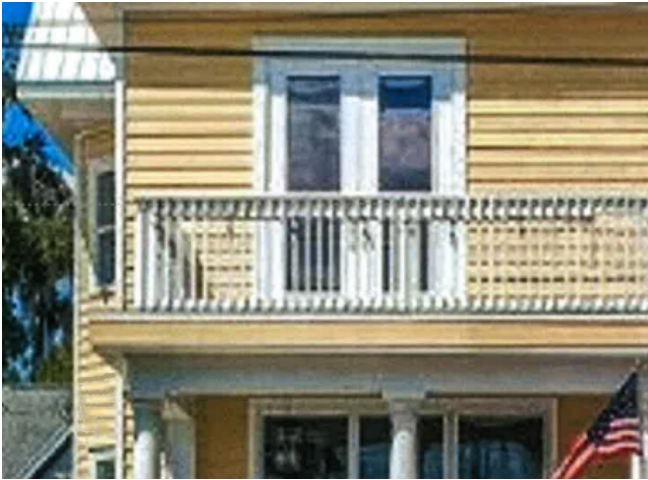
Figure 4 Photograph of the existing door and balcony/railing on the single-family dwelling at 414 River Street.
