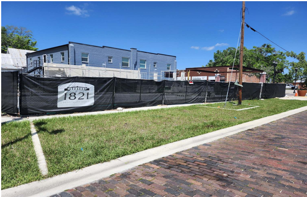
VIEW LOOKING AT THE EASTERN BORDER OF PARCEL B FROM S. 8 TH STREET (The proposed easement is located along this sidewalk)
