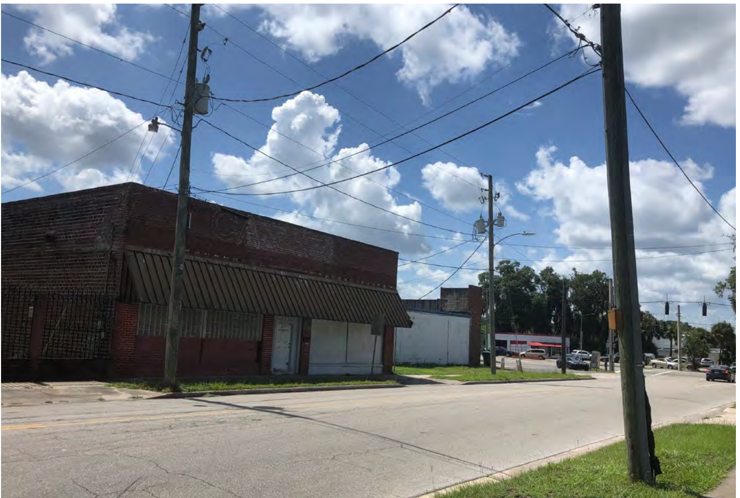
Image 9 Vacant Building in Palatka, FL
