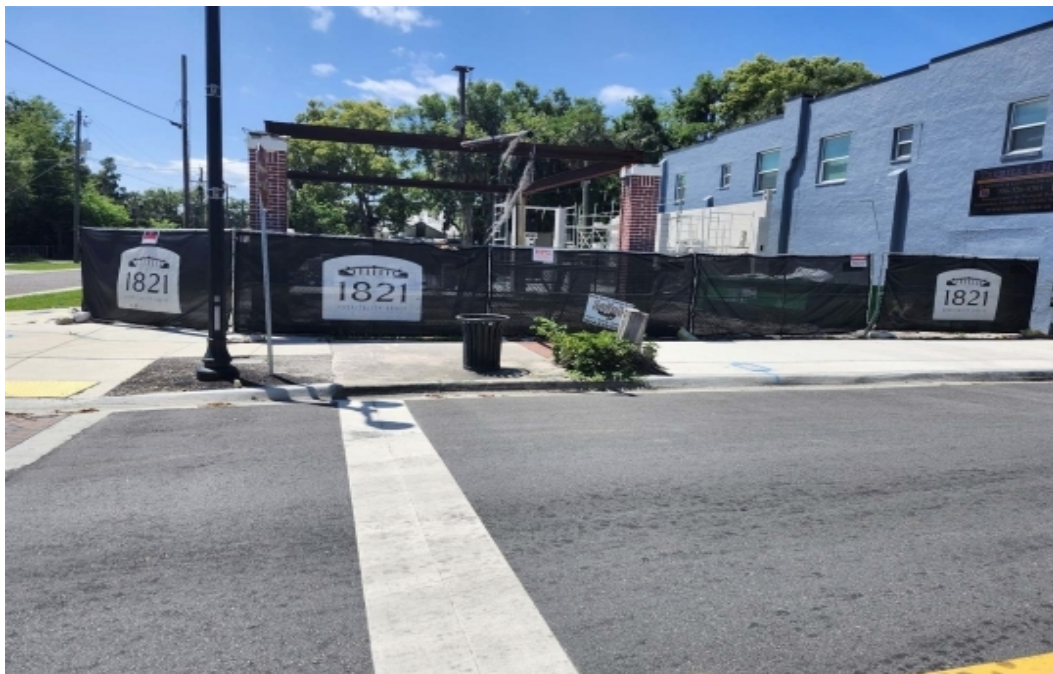
VIEW LOOKING AT PARCEL B FROM ST. JOHNS AVENUE
