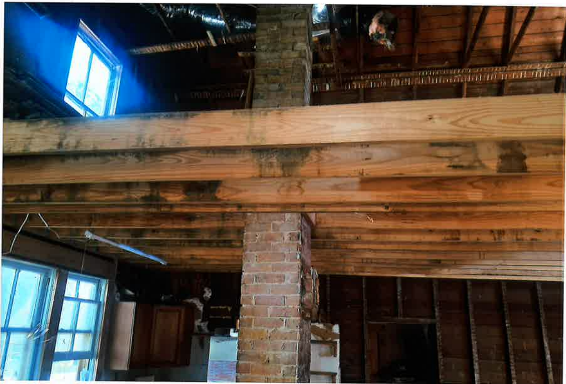
NEW 2 ND STORY JOISTS REAR
