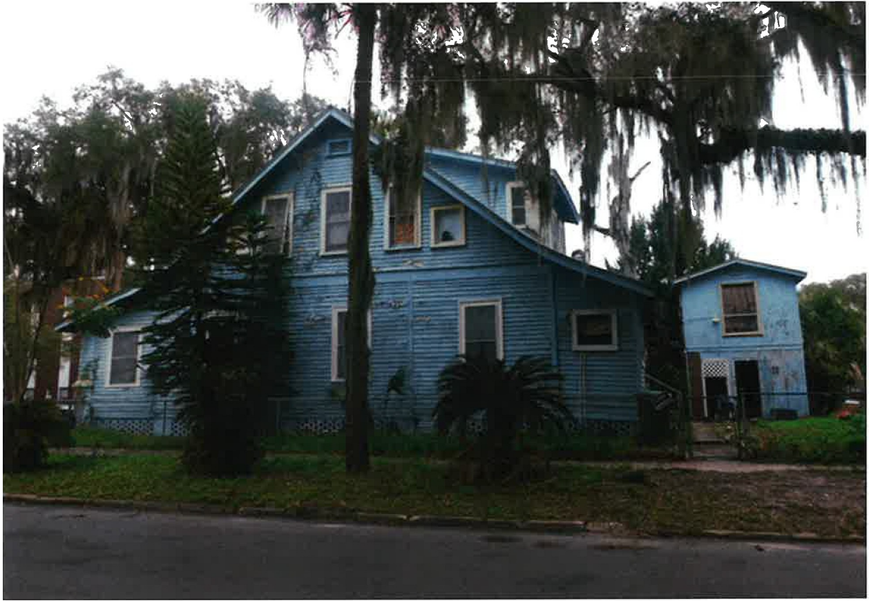
Before photo of house and shed.
