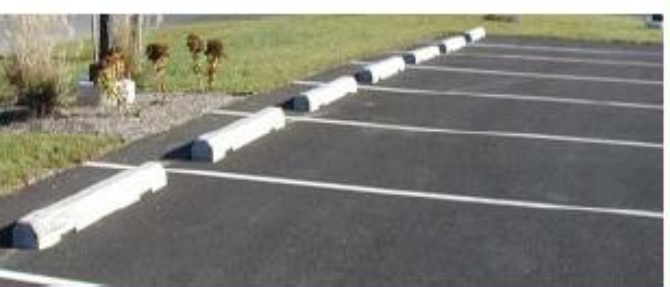
Grass island with parking stops on each parking space surrounding the island (no curb required on island)
