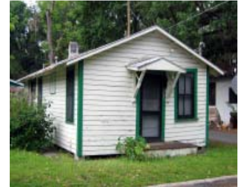
Avoid removal of features that form the historic character of a building. Repair if possible, or replace if necessary.
