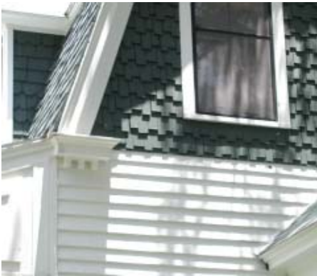
The exterior fabric of the Matheson House exhibits cypress shingles at gable ends and horizontal wood lap siding on first level.
