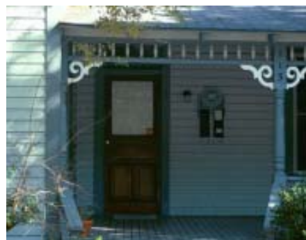
Decorative wood scroll detail on residence in Southeast District.
