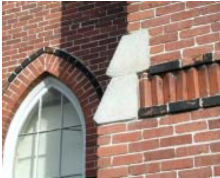
Detail showing stone used in combination with brick in Northeast District.
