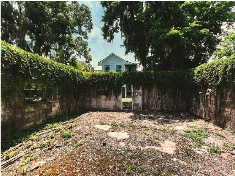
Figure 5 Remnants of a concrete structure located in the rear of the property.
