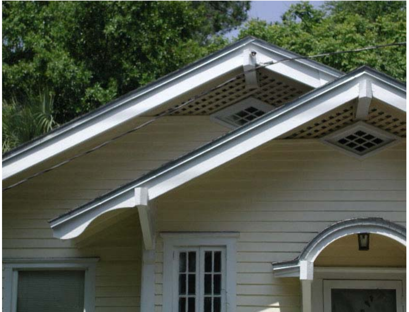
Eave detail of exposed rafters and gable vent of small wood frame Craftsman/Bungalow style house.
