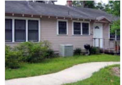
Mechanical systems should not be placed in front yards.
