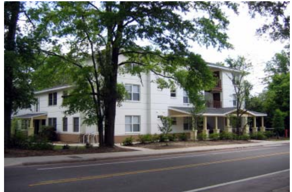
3-story addition on 2-story historic structure in University Heights South District
