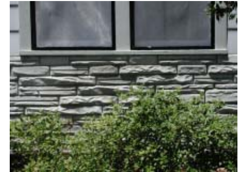
Fieldstone at base of residence.
