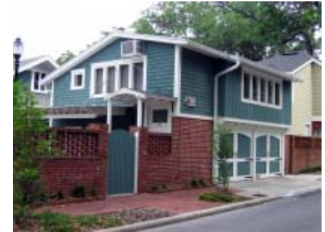
Rehabilitation of a garage apartment in the University Heights North District
