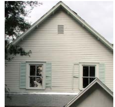
Repairs are warranted when required by the physical condition of character-defining materials and features.
