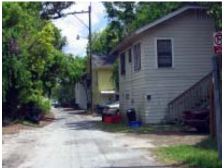
Retain landscape features such as streets, alleys, and setbacks that have traditionally linked buildings to the environment.
