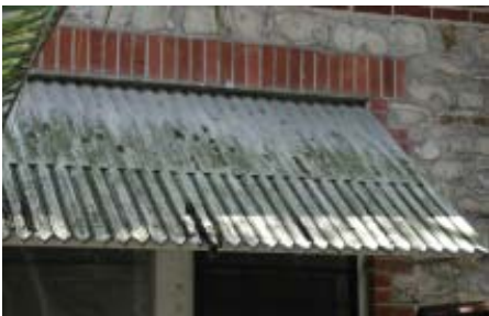
Awning on residence in Southeast District.
