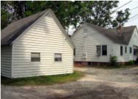
Auxilliary structures should use materials similar in size, proportion and detail to the principal structure.
