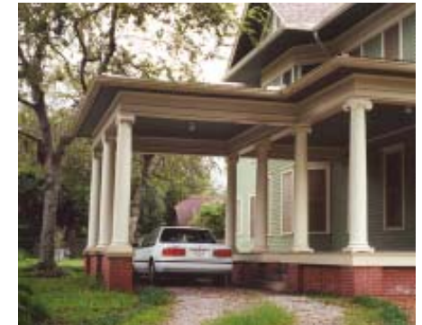
Porte cocheres and garages are often an integral part of the original design of historic buildings.
