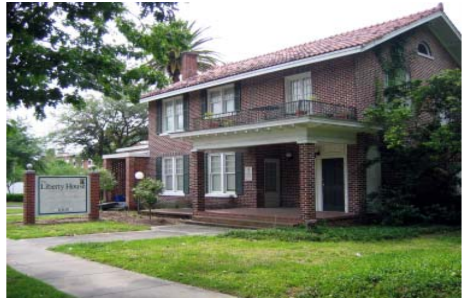
Rehabilitation project on SW 2nd Avenue.
