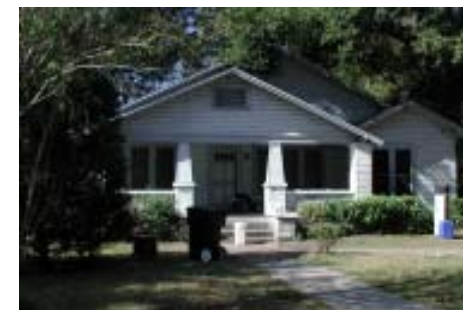
Bungalow style house in Pleasant Street District.
