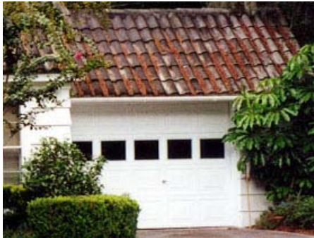
Clay tile roof tile in Northeast District.
