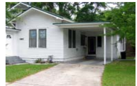
Carport in the University Heights North District.
