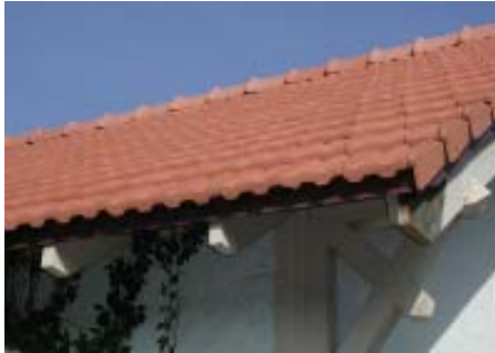
New synthetic roof tile representing historic material.
