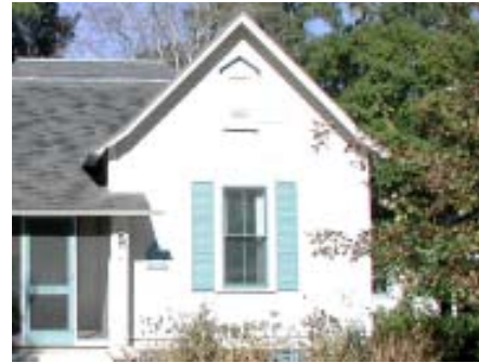
Window shutters on residence in Northeast District.
