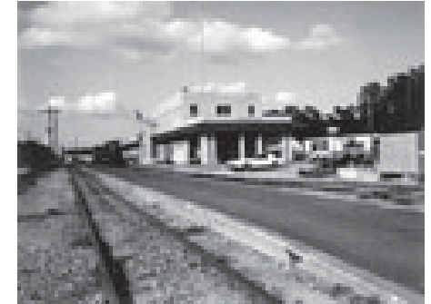
Train station on 6th Street prior to renovation as Santa Fe Community College Downtown Campus.
