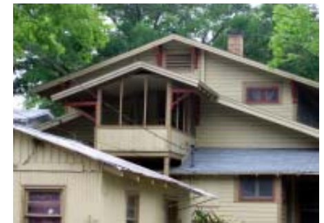
Complex roof form and multiple materials
