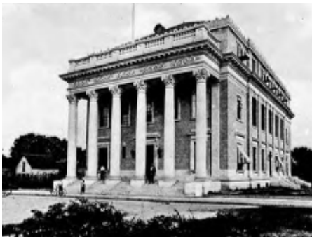
Elevation of the Beaux Arts style building.
