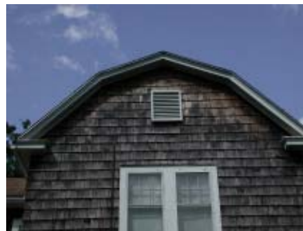
Wood shingles on residence in Northeast District.
