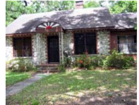
Fieldstone and brick construction in South District. Known locally as “chert” houses, the technique was used for a variety of historic styles
