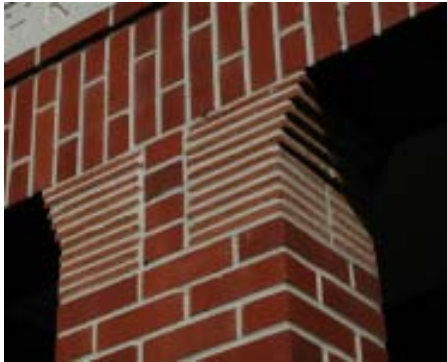
Brick detail at the First United Methodist Church, Northeast District.
