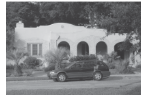
Elevation of a Mission style building in Northeast District.
