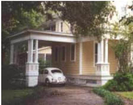
Porte cocheres and detached garages are visible expressions of the impact of the automobile on historic buildings in Florida.
