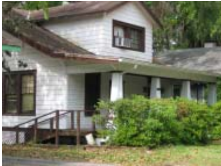
Ramps should not destroy character-defining qualities of the architecture.
