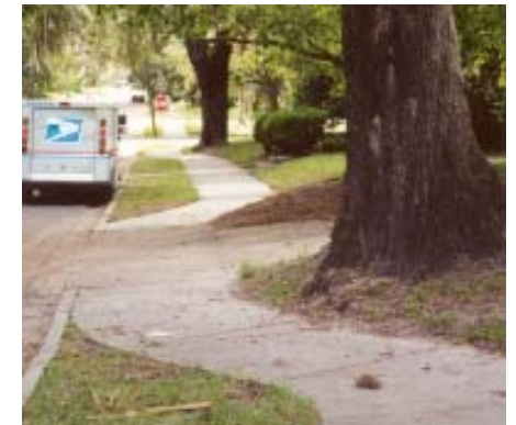
Existing sidewalks within the district should be maintained.
