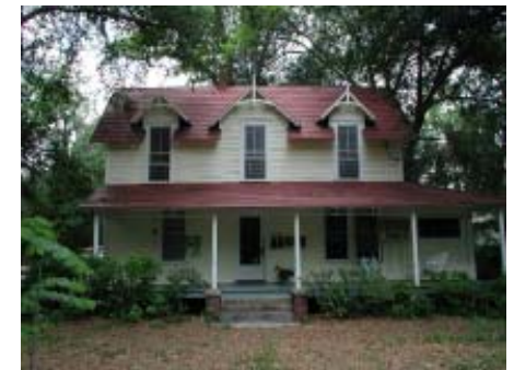
Elevation of the Gothic Revival style building.
