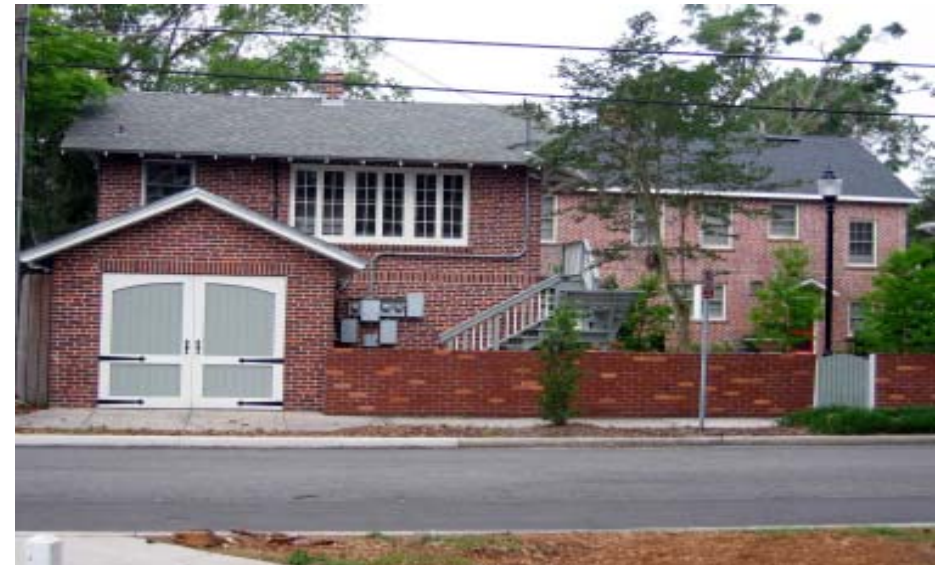
Auxilliary structures should use materials similar in size, proportion and detail to the principal structure.
