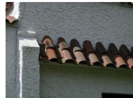
Detail of terra cotta tile above window.
