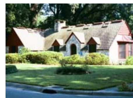
Massive stone walls of the Pierson House, Northeast District.
