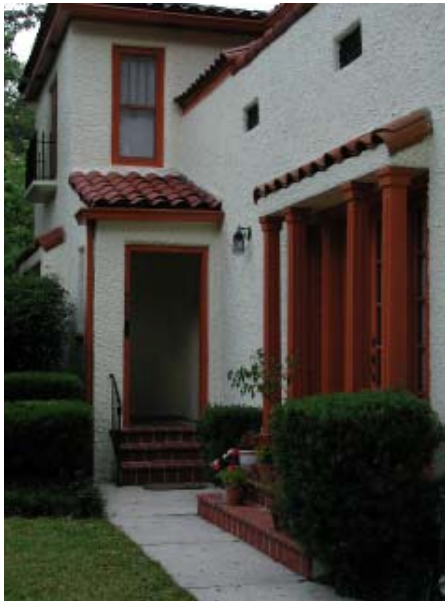
Textured stucco on Mediterranean style residence in Northeast District.
