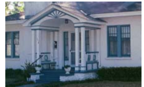
Entry porch with built in benches in Northeast District.
