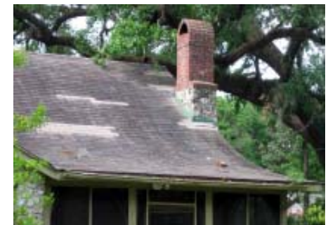
Retain distinctive architectural or stylistic features that give a roof its essential character.
