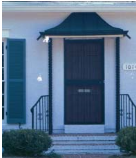
Ornamental metal entry roof, Northeast District.
