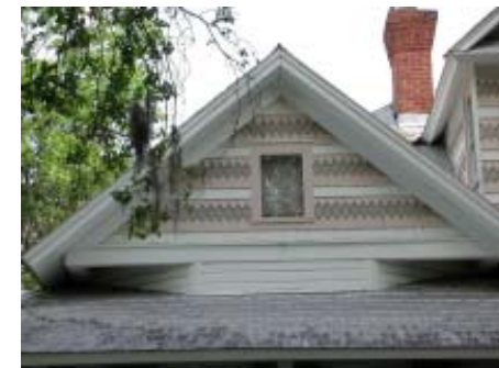
Decorative wood shingles on gable end of residence in Northeast District.
