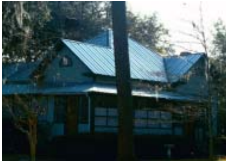
New metal roof, Northeast District.
