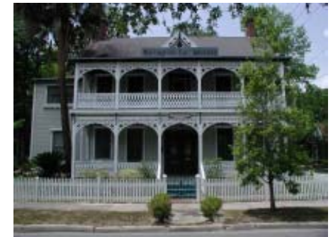
A proud example of another renovation project in Pleasant Street District is Warrington’s Fine Interiors.
