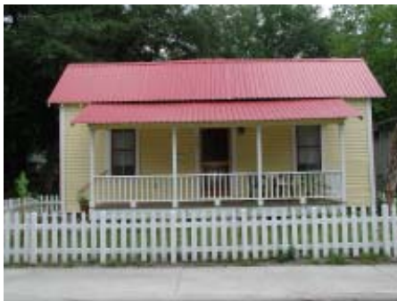
Over forty deteriorated structures have been restored within the District.
