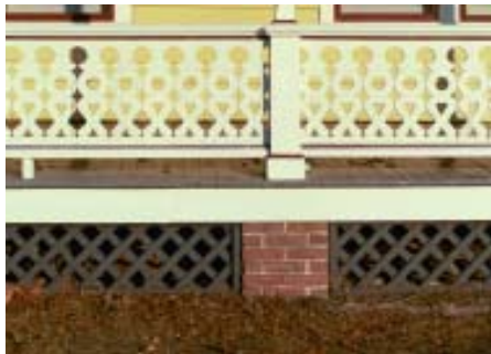
Lattice infill at pier foundation with pier expressed.
