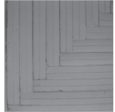
Detail of ceiling on porch of the Medlin House, Southeast District.
