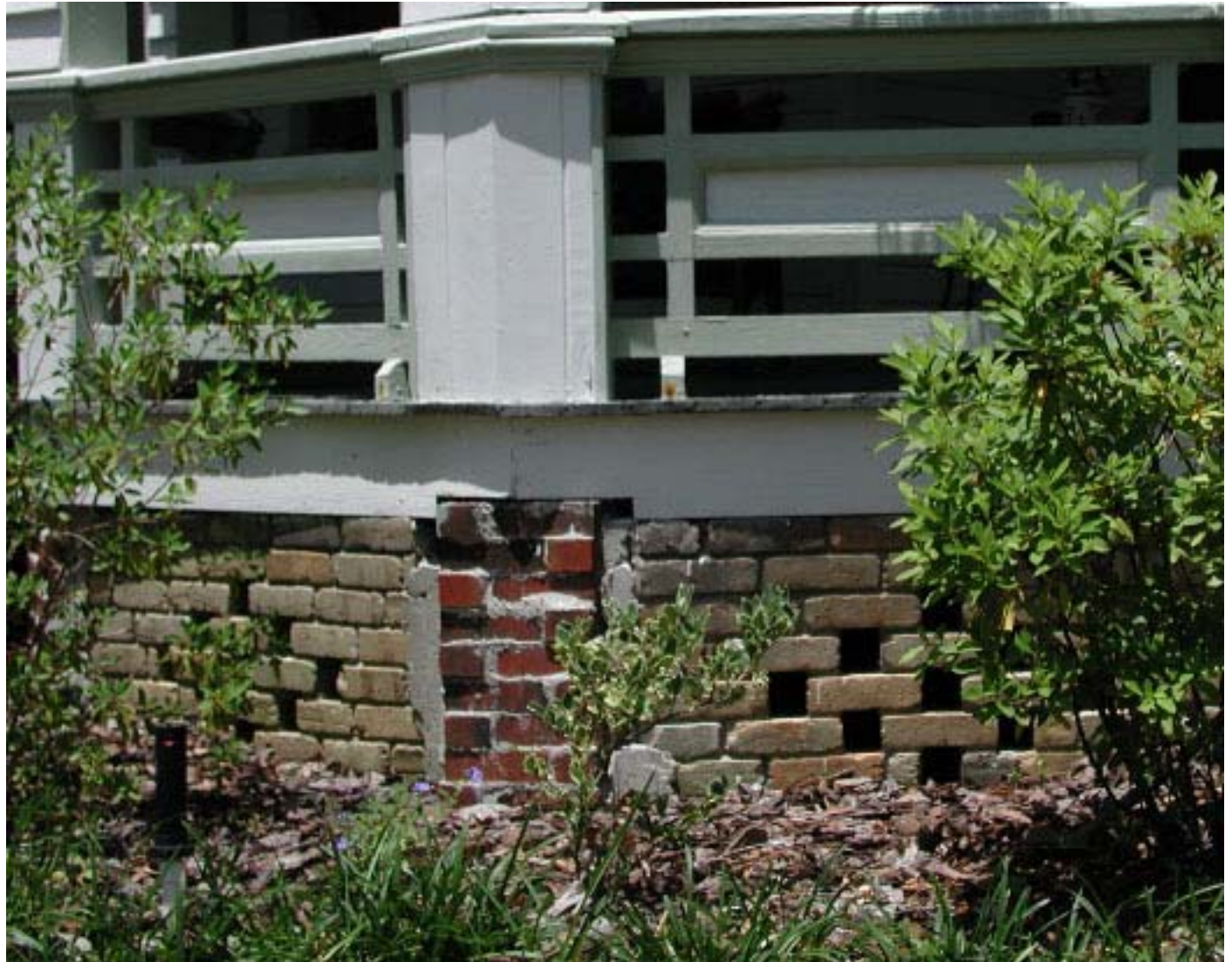
Foundation repairs, the historic materials should be retained, repaired as needed, or replaced with similar materials.
