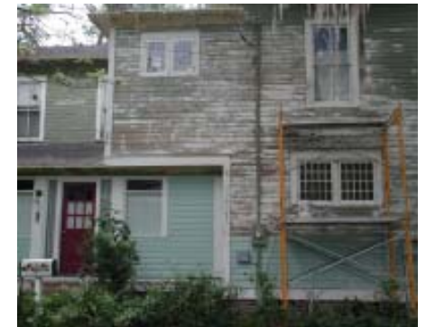
Restoration work done in the Northeast District.
