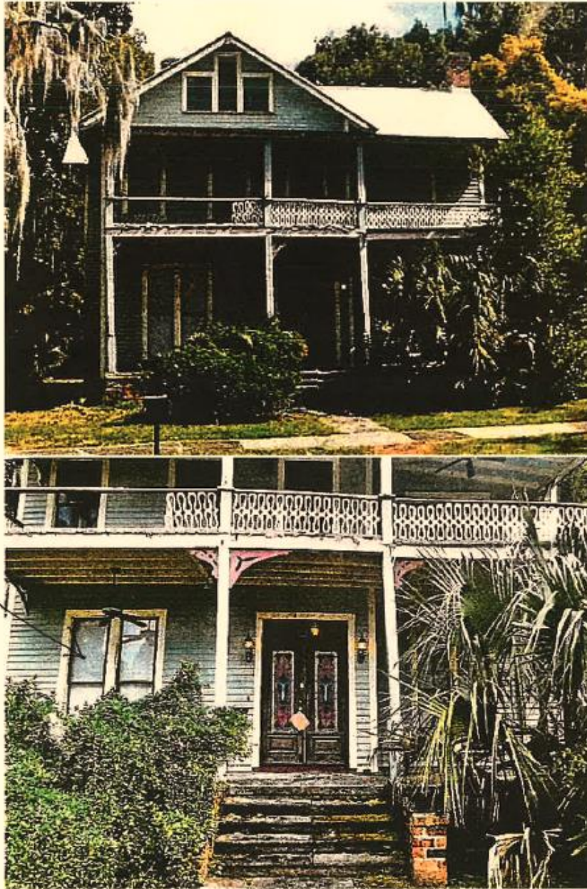
Figure 3. Photos before replacing the porch and railing of 417 N. 3rd St.
