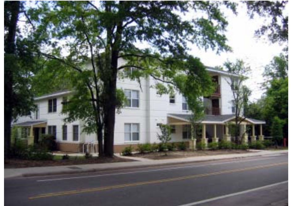
New 3-story addition to existing two-story structure with new pedestrian-friendly porches.
