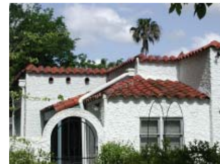
Terra cotta roofing tile and ornament exhibited on Mediterranean style residences in Northeast District.
