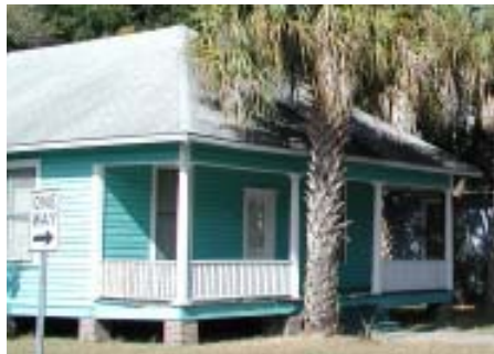
Simple porch detail of frame vernacular style residence in Pleasant Street District.
