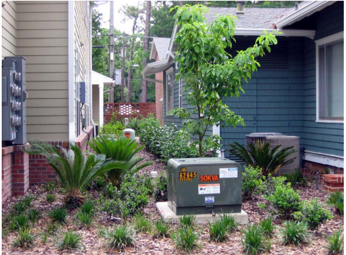
Mechanical systems should be screened from view.
