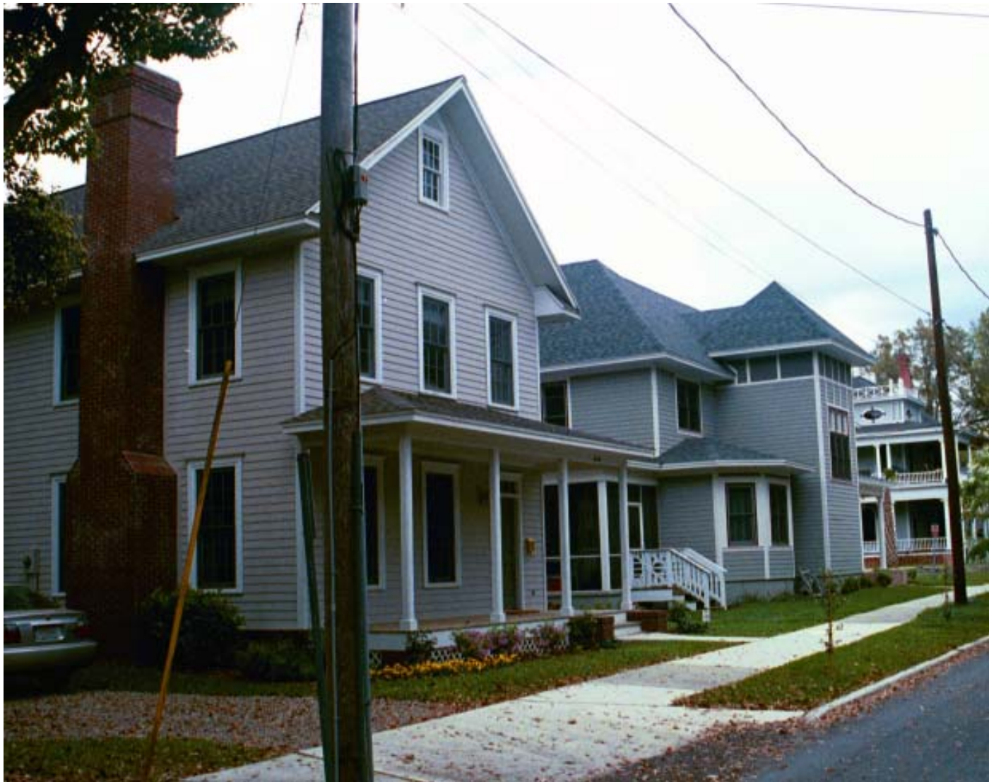
New infill construction in Northeast District.
