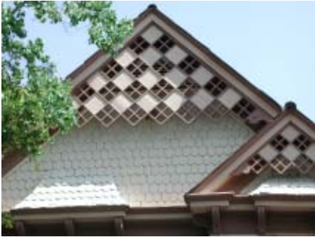
Decorative woodwork eave details at gable end of building.
