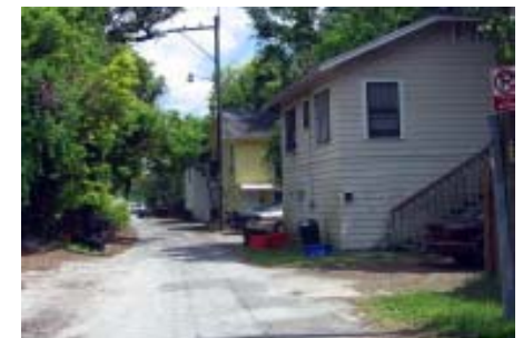
Garage apartments along mid-block alleyways in University Heights South District.
