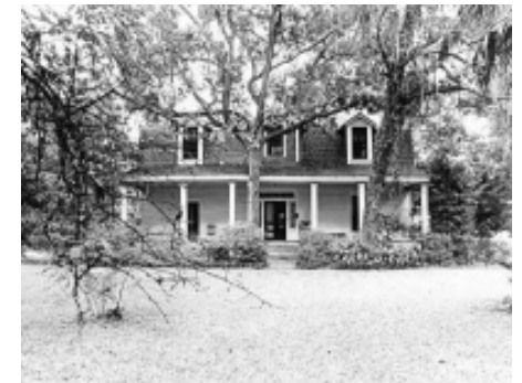
Matheson House is one of the oldest existing buildings in the Southeast District, c.19--.
