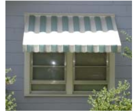
Awning on residence in Southeast District.
