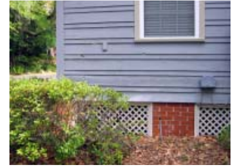
Wood lattice infill with brick pier.
