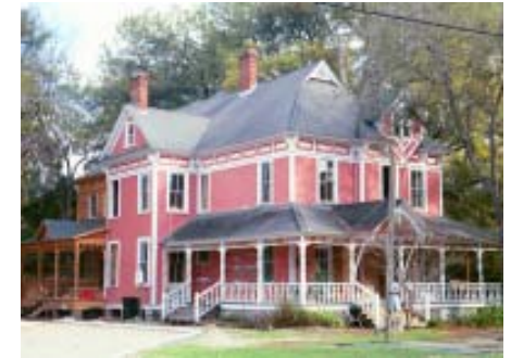
The renovation and rehabilitation of this historic building will soon open as Laural Oaks, a new Bed and Breakfast on S.E. 7th Street.
