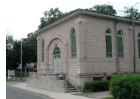
Rusticated concrete block utilized on the Friendship Baptist Church, Pleasant Street District.
