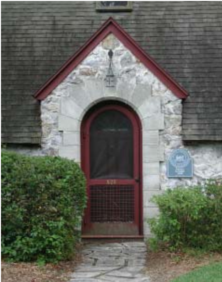
Detail showing stone and chert rock entry on Pierson House in Northeast District.
