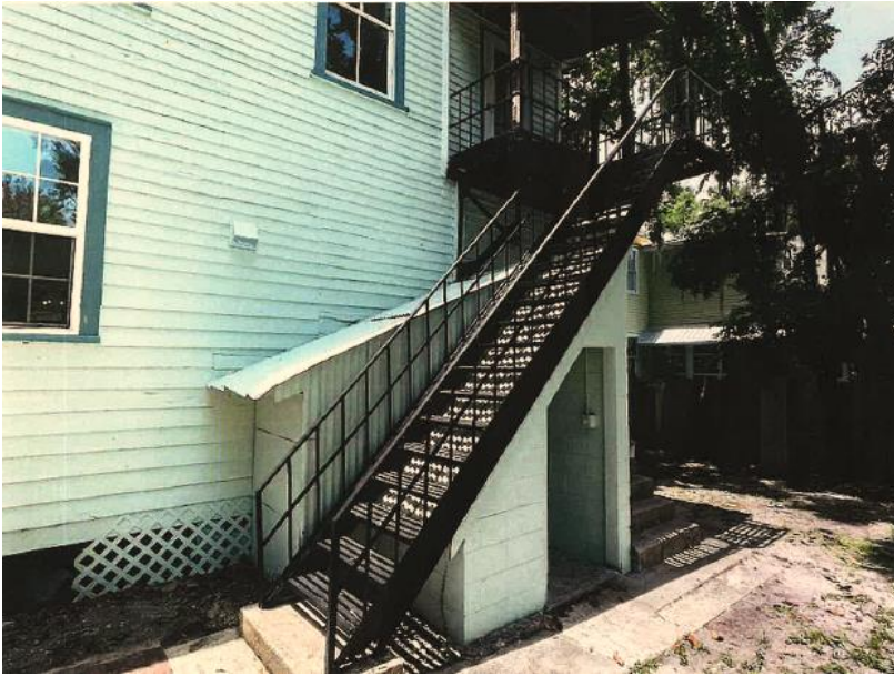
Figure 4 View from the East, rear of the house, showing metal staircase and storage area to be removed.
