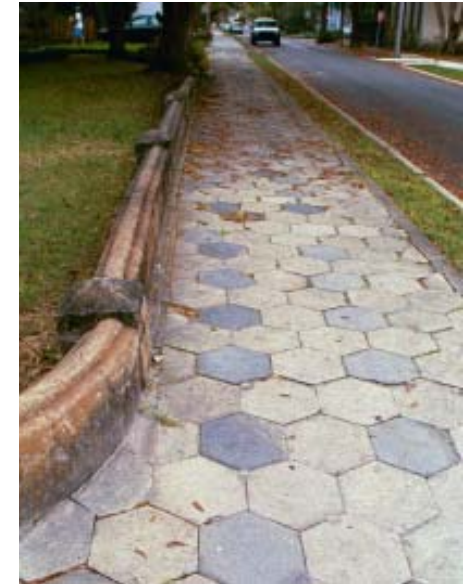
Identify and retain curbing, fencing, walkways, street lighting, signs, and benches that reflect a property's history and development.
