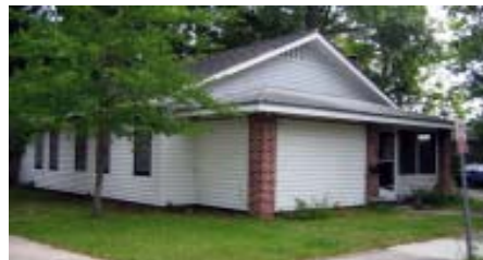
Enclosing a porch or porte cochere radically changes the appearance of the principal building.
