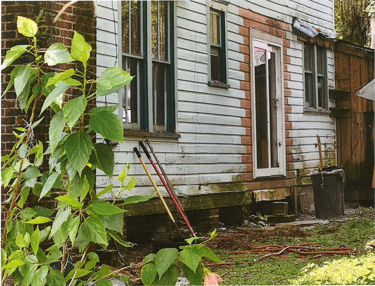
Figure 5 window replaced Pella Impervia Series 75" X 80" X 5 5/8" Jamb Brown fiberglass $3454.95 and,proposed stair area.
