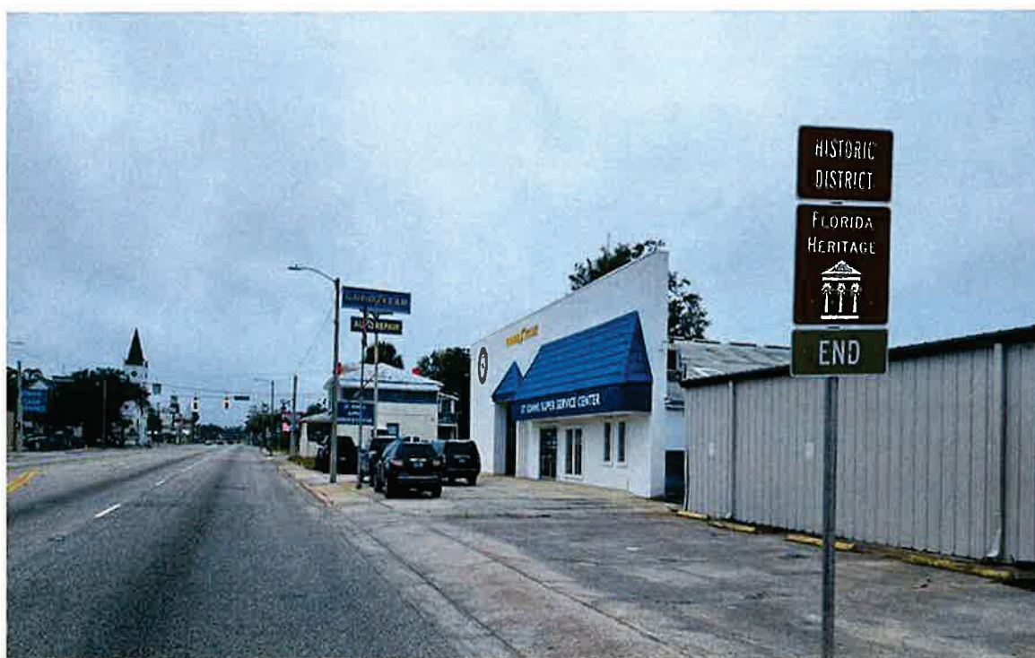
(6) St. Johns Super Service Center - 608 Reid Street – Vehicle repair shop
