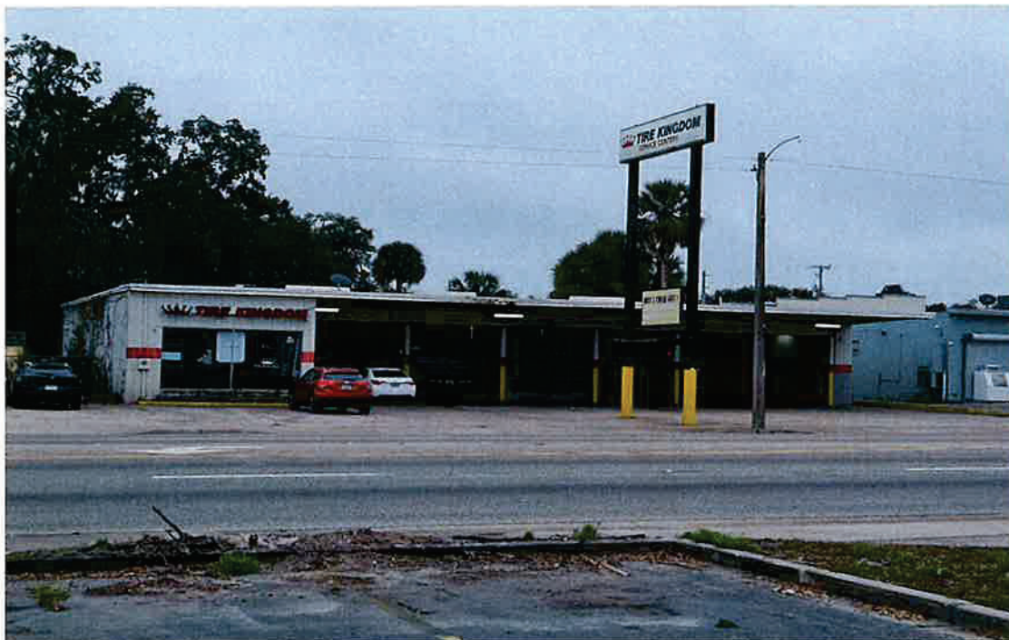
(1) Tire Kingdom - 813 Reid Street - Auto repair shop across the street from 820 Reid Street
